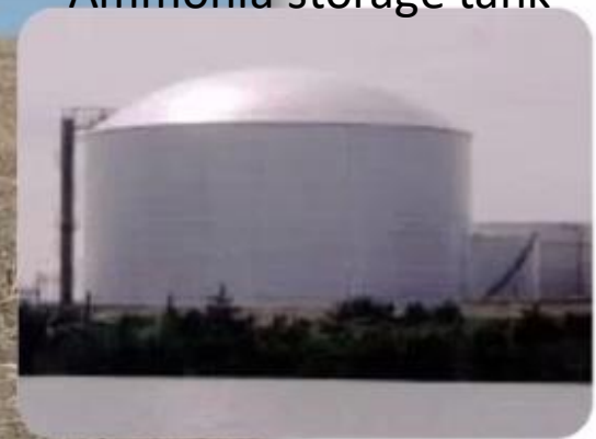
Ammonia storage tank
